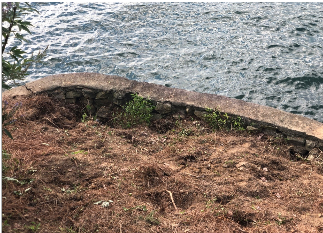
Figure 3-4. Erosion of soils from behind bulkhead on Lake Burton
